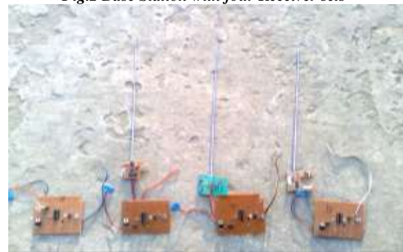
Fig.3 Four Sensing units with individual Transmitters
